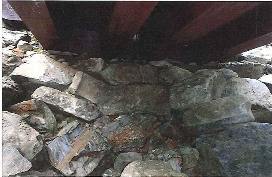
CK2319 Right Abutment
