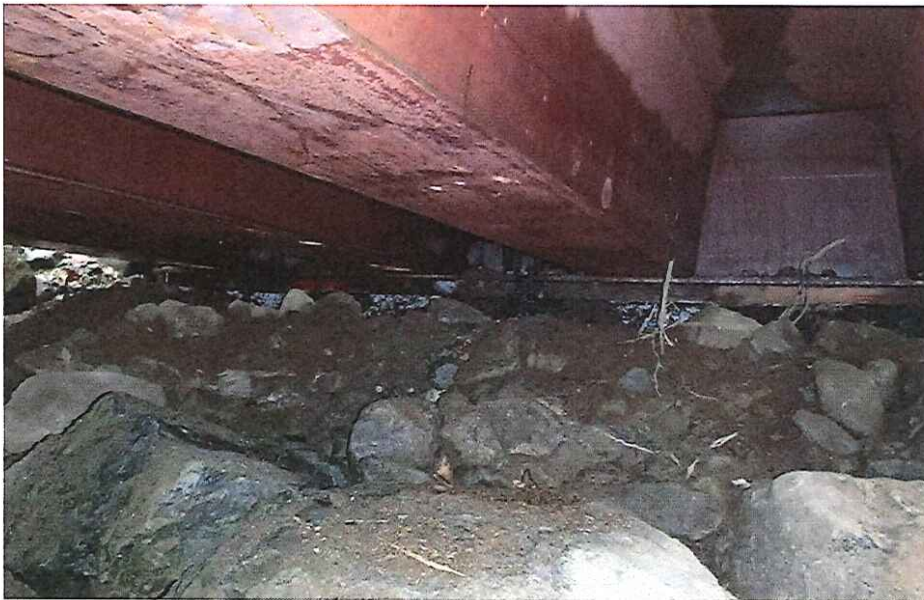
CK2319 Left Abutment
